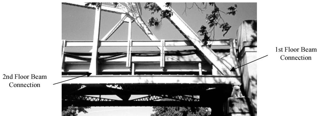
Figure 4.13 Floor Beam to Truss Connections
