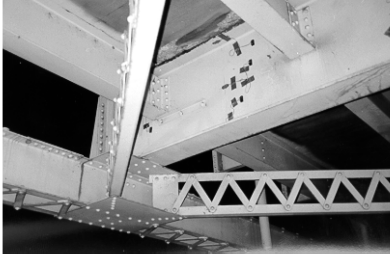
Figure 4.3 Connection of Second Floor Beam to Truss
